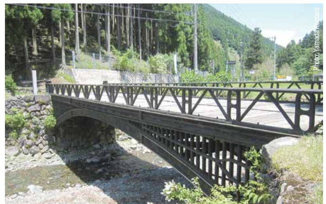
The Mikohata Bridge built in 1885 (Asago City, Hyogo Prefecture)
